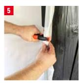
Finally, the protruding foil must be attached to the drywall supports. To do this, use adhesive tape or, as shown in the picture, spring clamps that can be fixed quickly.
