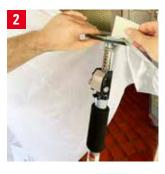
Fix the foil with the help of an adhesive tape on the upper support surface of the drywall support.
