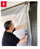
As soon as the drywall support stands vertically between the ceiling and the floor, turn the handle clockwise to fix the support
