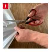
Cut the foil to the required size. Note a foil overhang of approx. 10 cm per side.
